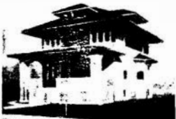
A No. 100 IDEAL Boiler and 600 ft. of 3/4" AMERICAN Radiators, costing the owner $255, were used to Heat Water in this house.
